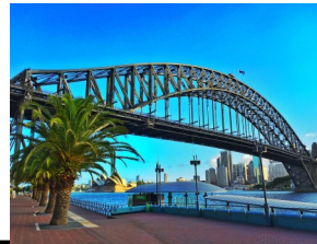
Sydney Harbour Bridge
